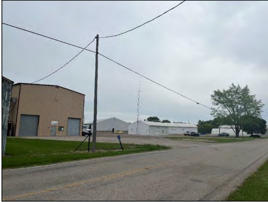
Photograph 3. Mercer Landmark – Convo Agronomy, located at 5703 Convo Road, is an industrial development located within the study area.
