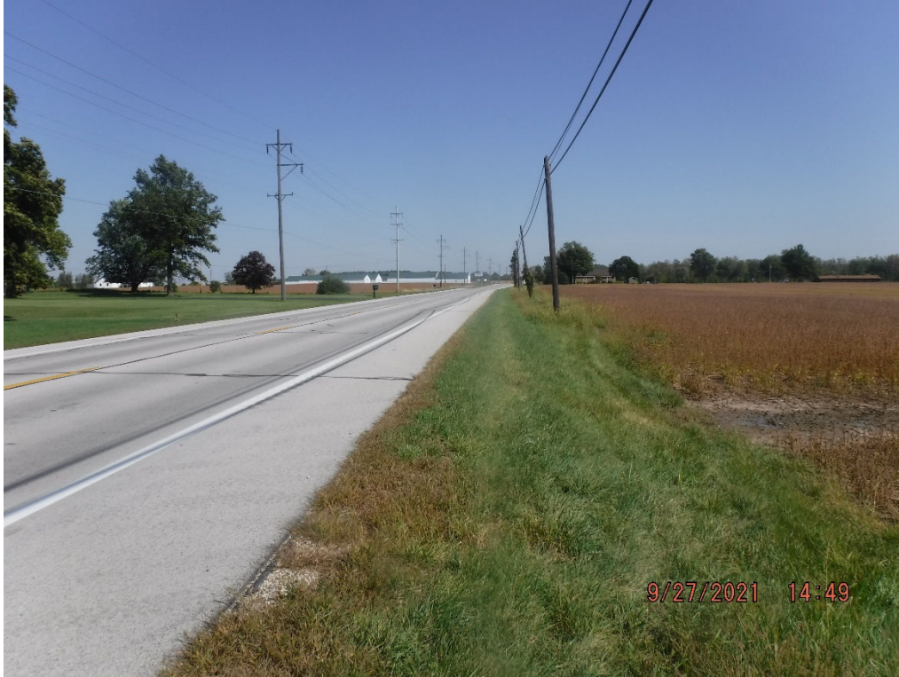
Photo 1. Road right-of-way (ROW) along S.R. 703 within the western portion of the project area.
