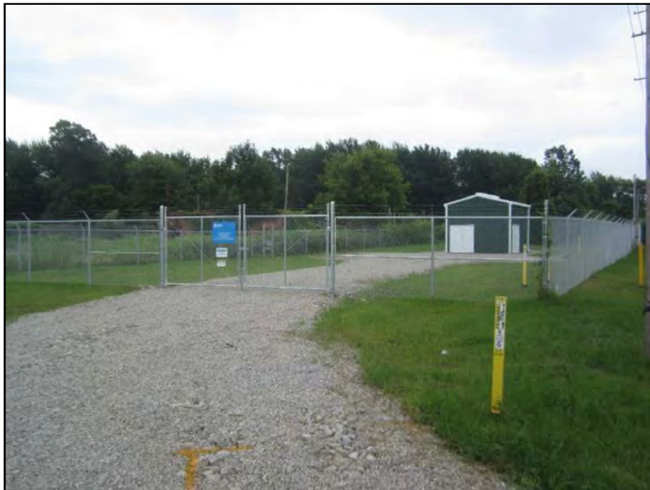
Photograph 4. A public utility development is located south of West 30 th Street within the eastern portion of the project area.
