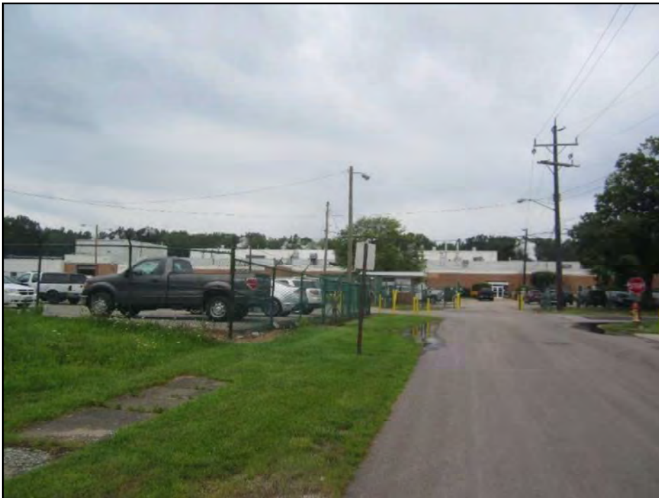
Photograph 2. Molded Fiber Glass Company, located at 2925 Mfg Place, is an industrial development located within the project area.
