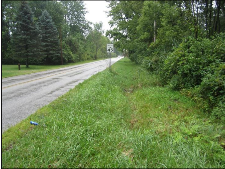
Photograph 5. Roadside ditches are located along Wade Avenue within the study area.
