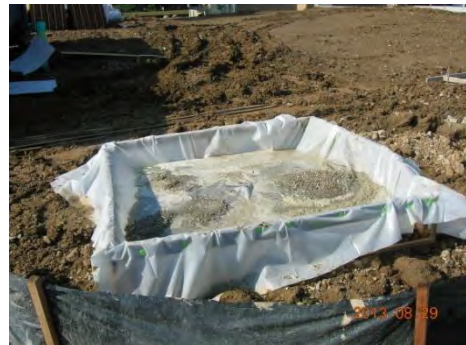
Photograph of the "ABOVE GRADE" concrete washout structure
