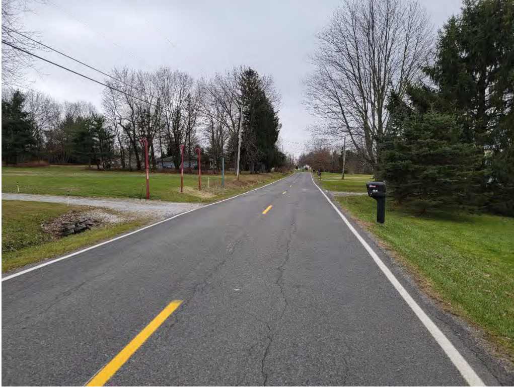
Photo 3. Road right-of-way (ROW) along Grove Road within the project area.
