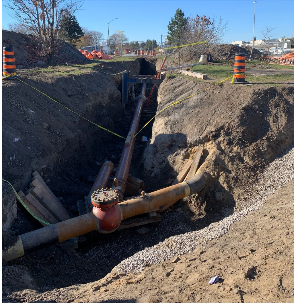
East Tie-in During my Visit on Nov. 2
