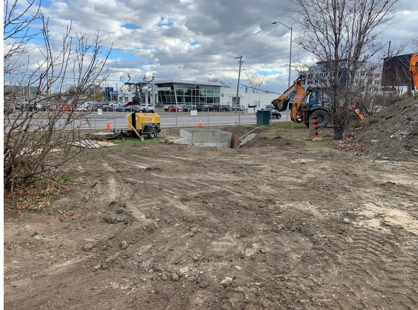
Same East Tie-in Site on Nov. 7
