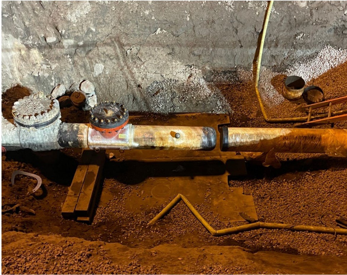
Cut and Cap West End (from On-ramp) – Nov. 9
