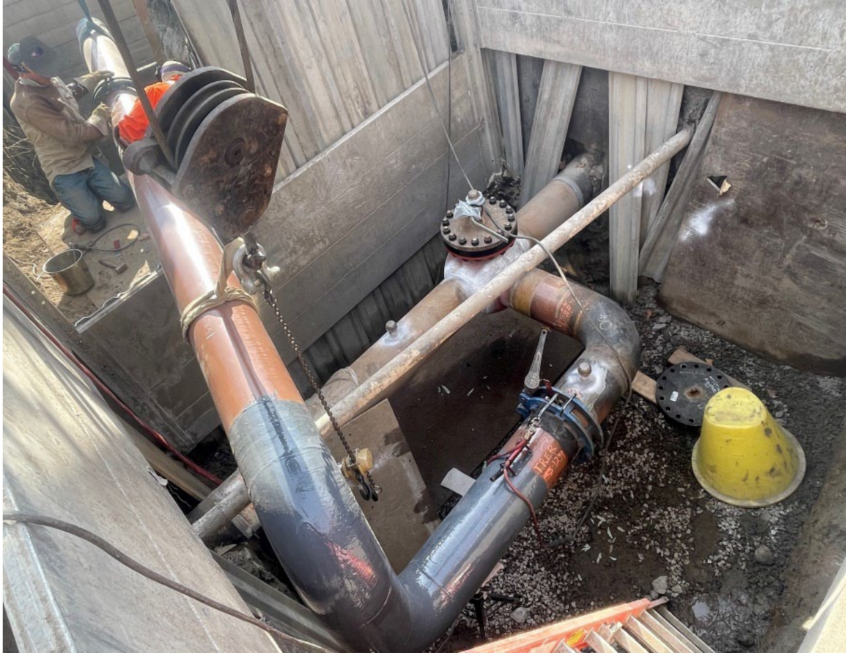
Weld being Completed near Tie-in Location (Earlier this Week)
