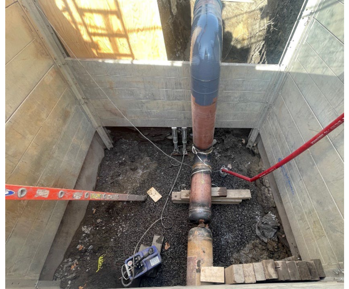
Final Tie-in Location (Earlier this Week)
