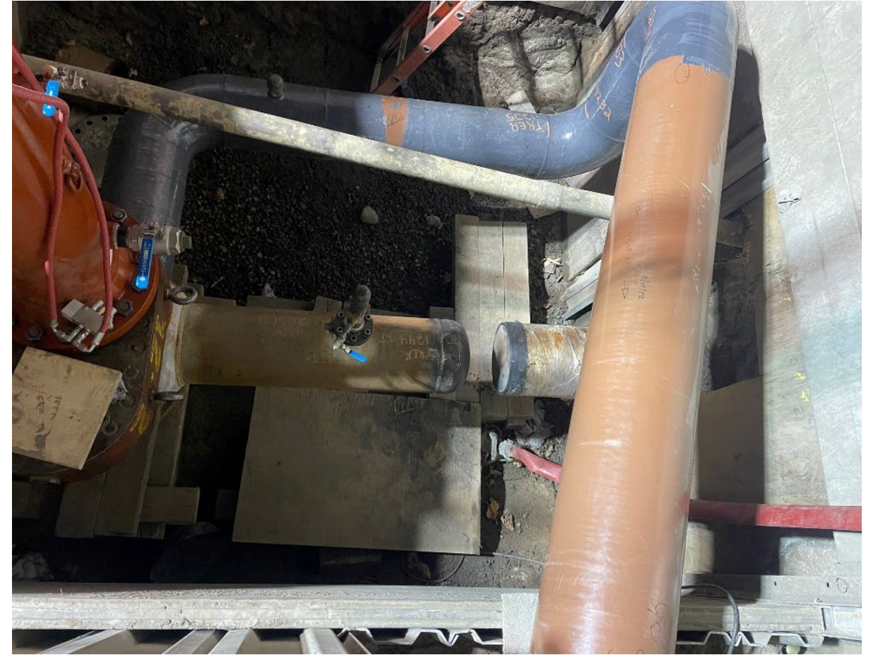
Cut and Cap East End (from On-ramp) – Nov. 9
