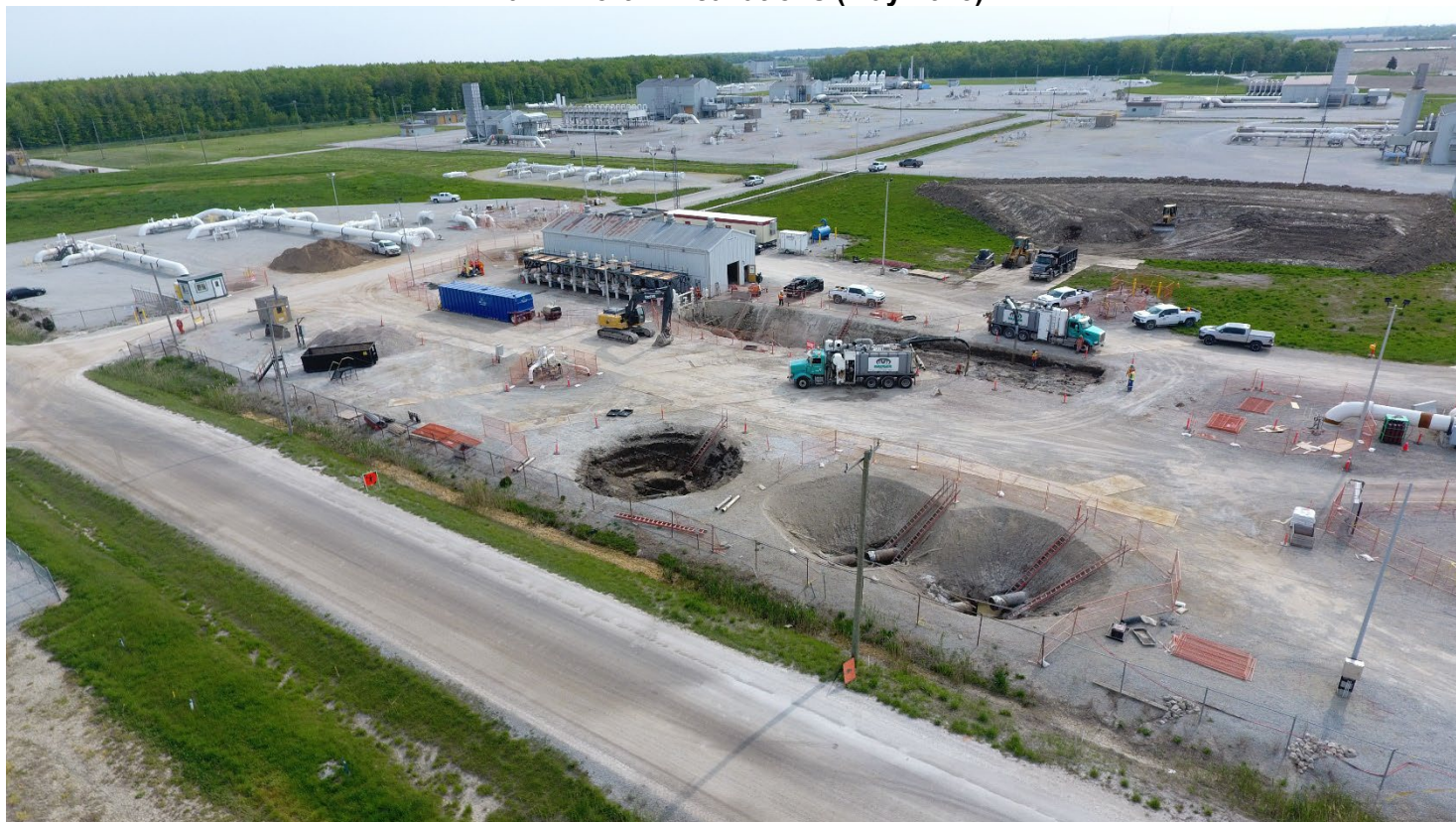
Dawn North Excavations (May 2023)
