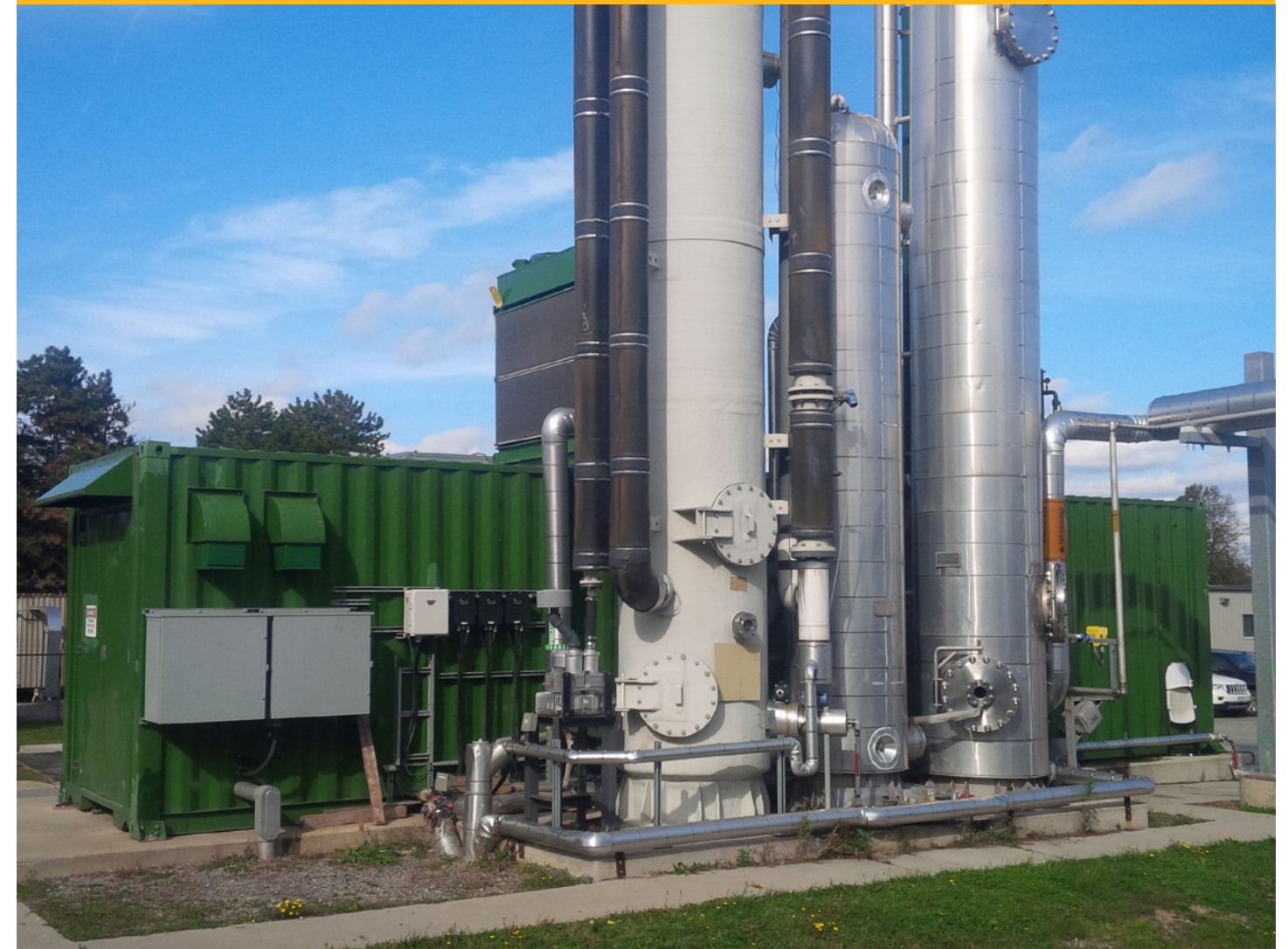
Hamilton Water Treatment Plant
