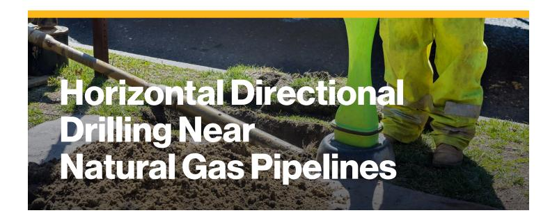
Horizontal directional drilling (HDD) or directional boring is a steerable trenchless method of installing underground facilities.
