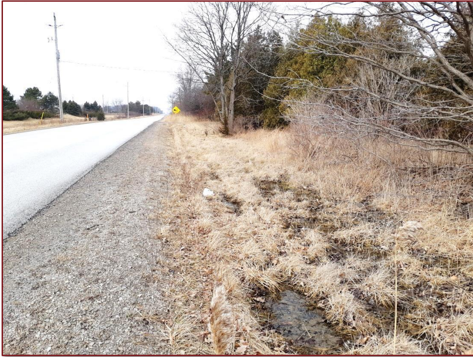
Image 24: Erieau Road ROW – Ditched
