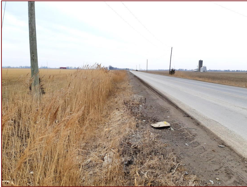
Image 32: Drury Line ROW – Ditched and Above Ground Utilities
