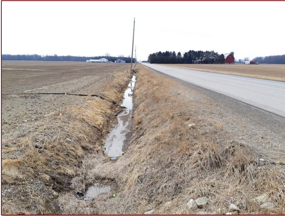
Image 40: Drury Line ROW – Ditched and Below Ground Utilities
