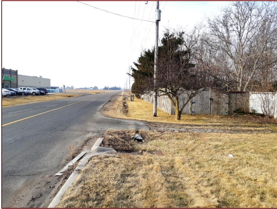
Image 4: Allison Line ROW – Ditched and Above Ground Utilities
