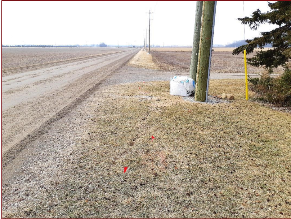
Image 18: Allison Line ROW – Ditched and Above Ground Utilities
