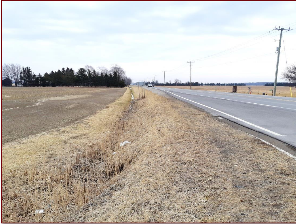
Image 54: Communication Road ROW – Ditched and Above Ground Utilities
