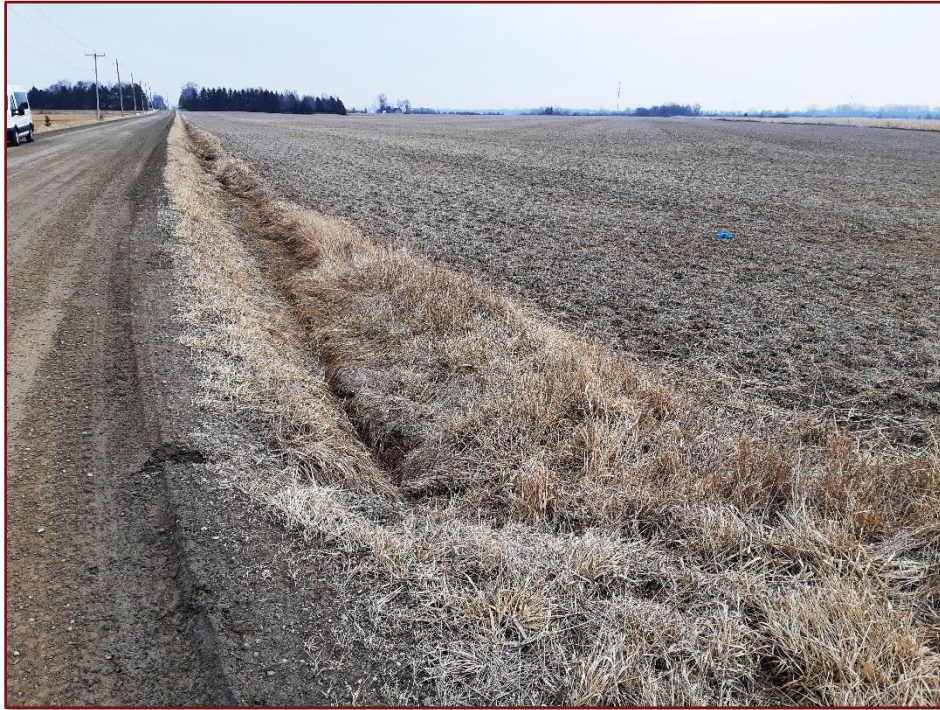
Image 20: Erieau Road ROW – Ditched and Above Ground Utilities
