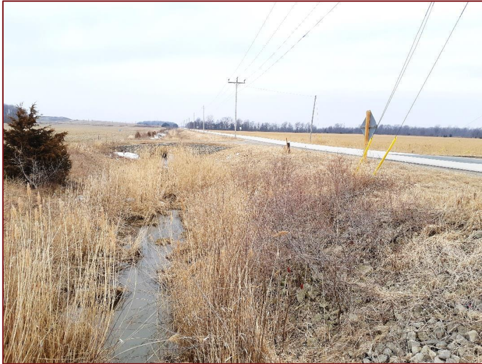
Image 22: Erieau Road ROW – Ditched and Above Ground Utilities
