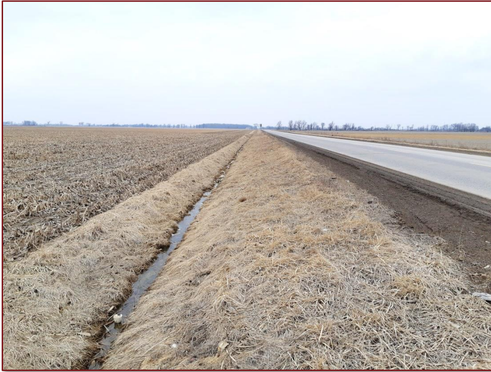
Image 28: Erieau Road ROW – Ditched
