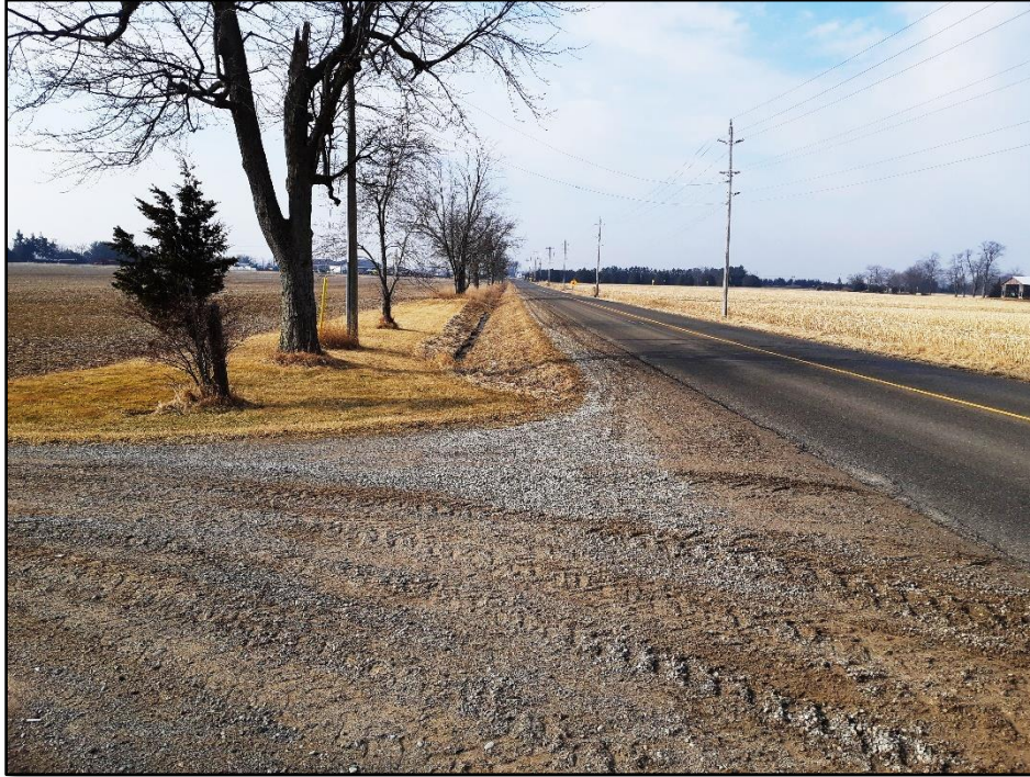
Image 6: Allison Line ROW – Ditched and Above Ground Utilities
