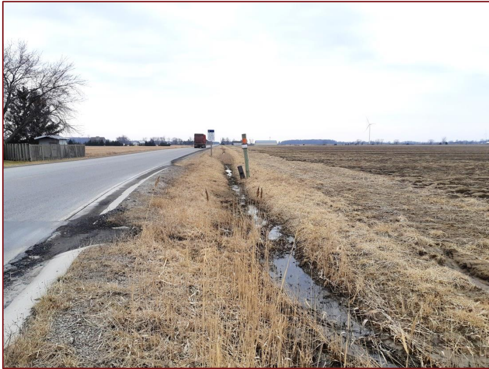
Image 46: Drury Line ROW – Ditched and Below Ground Utilities
