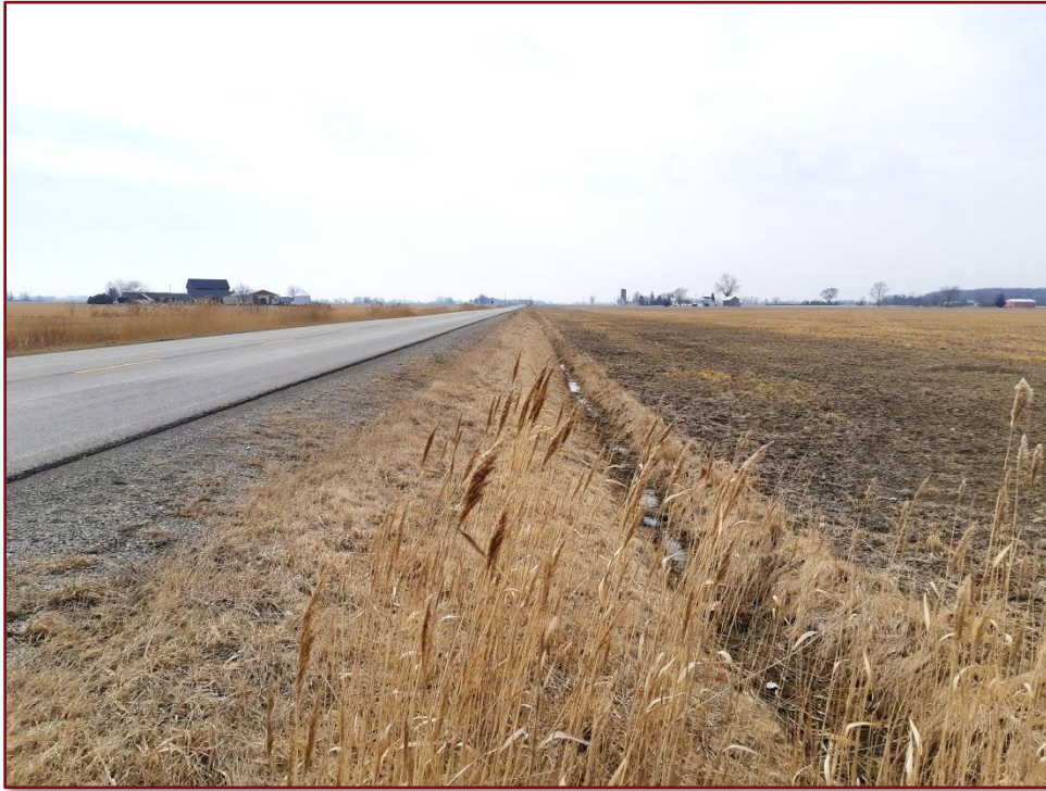
Image 36: Drury Line ROW – Ditched
