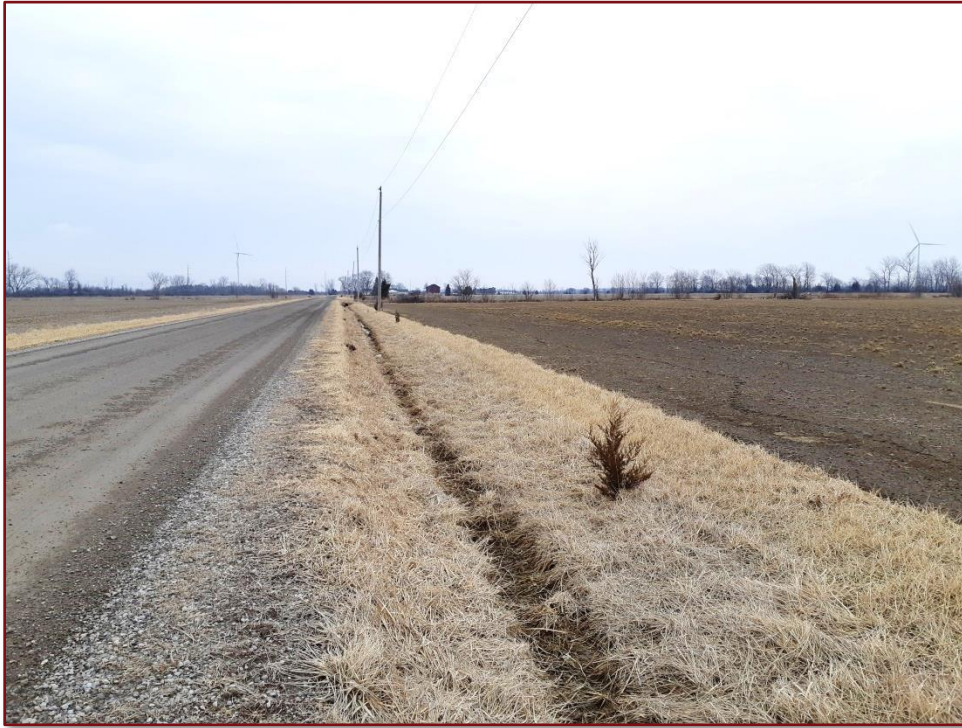
Image 50: Drury Line ROW – Ditched, Above and Below Ground Utilities
