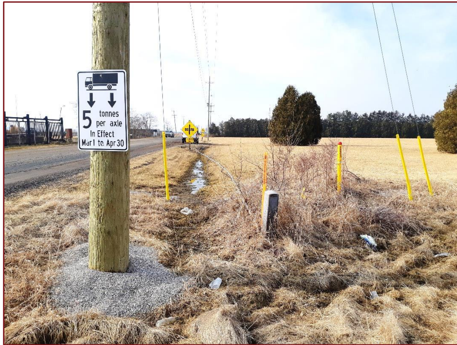
Image 8: Allison Line ROW – Ditched and Above Ground Utilities
