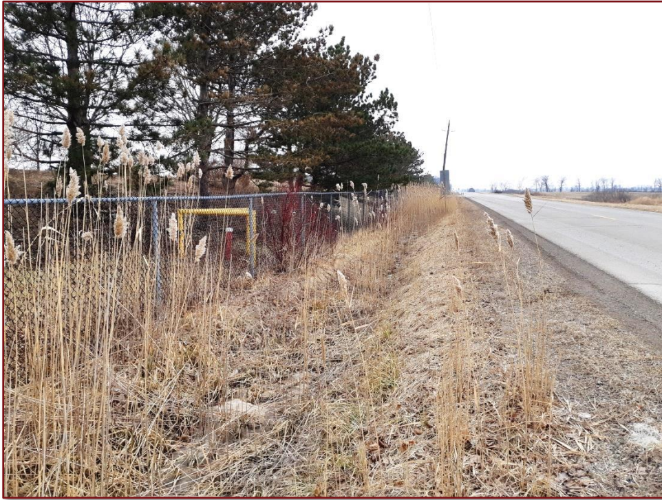
Image 26: Erieau Road ROW – Ditched
