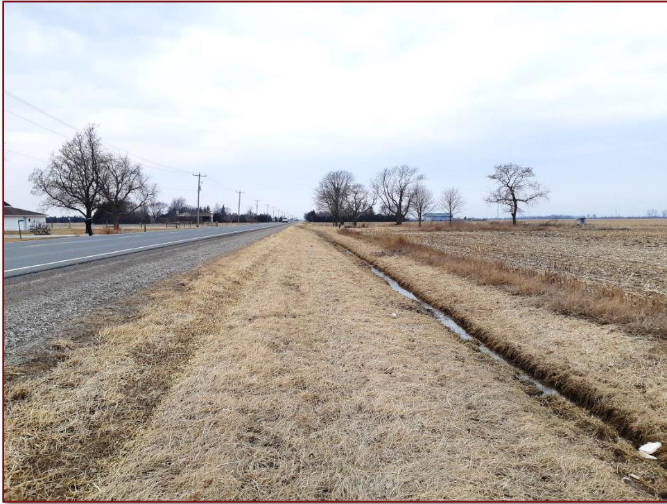
Image 58: Communication Road ROW – Ditched and Above Ground Utilities
