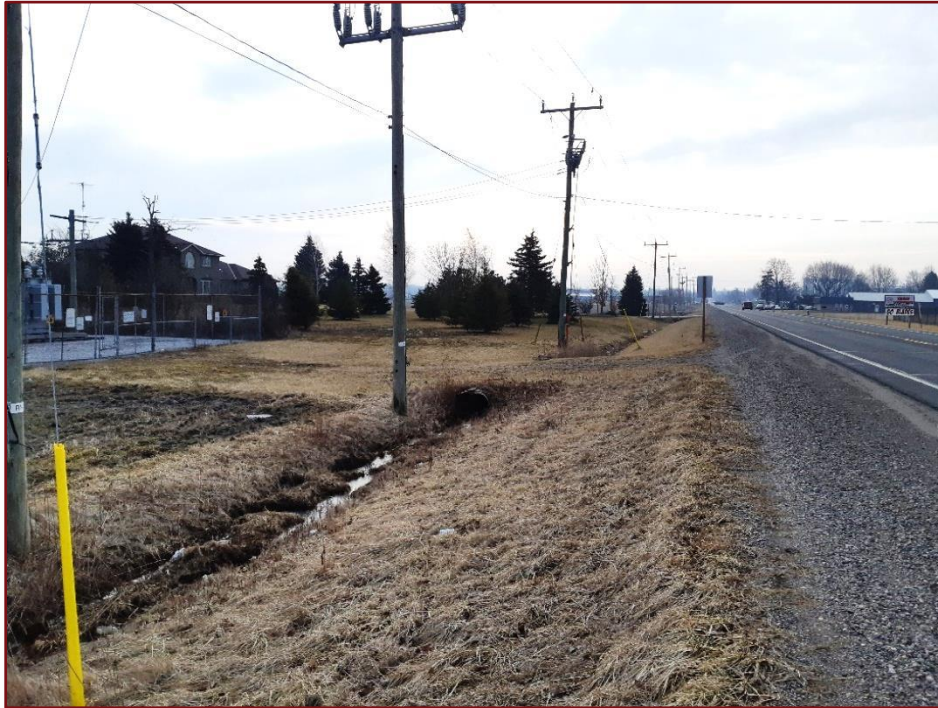
Image 2: Communication Road ROW – Ditched and Subsurface Utilities
