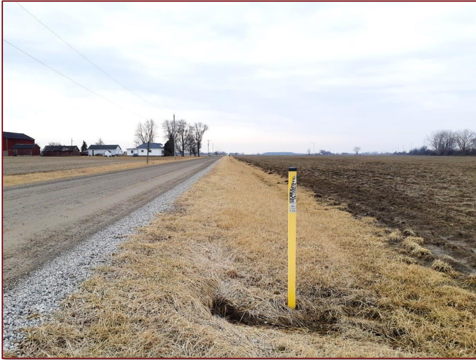
Image 52: Communication Road ROW – Ditched and Above Ground Utilities
