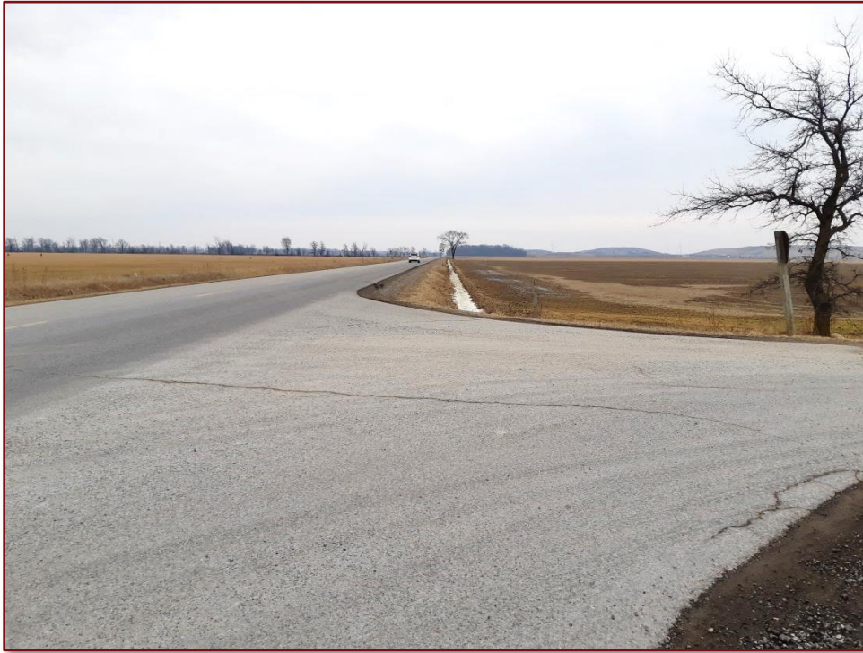
Image 30: Drury Line ROW - Ditched
