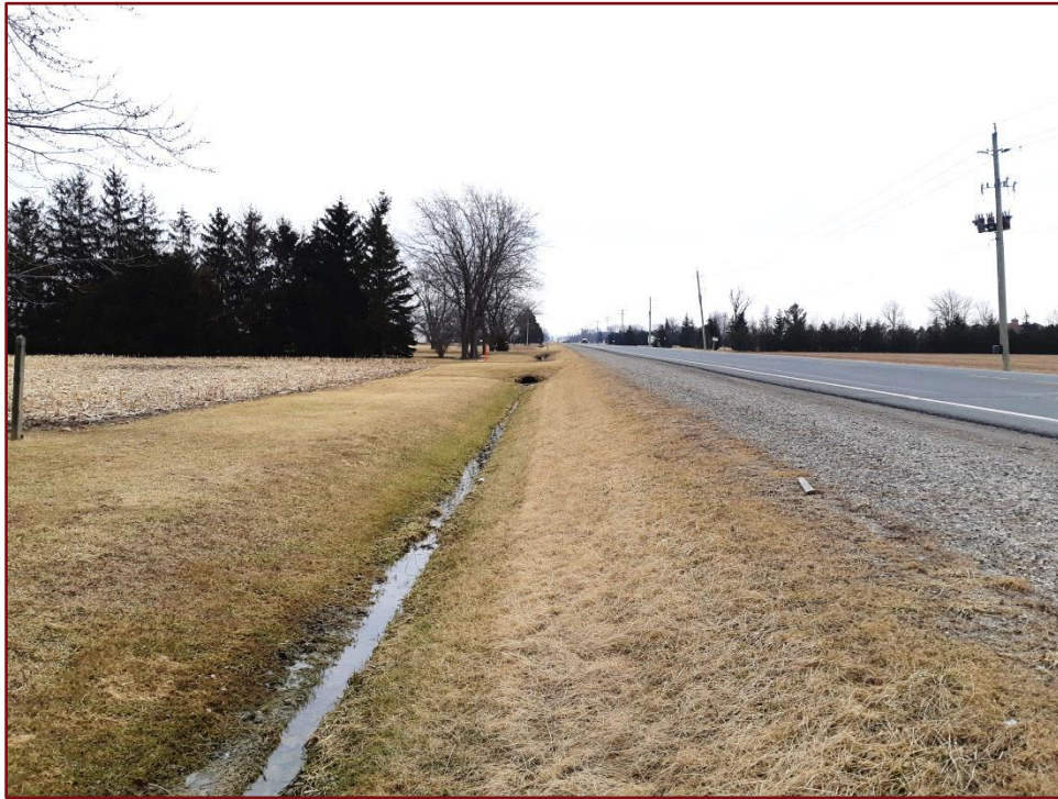
Image 56: Communication Road ROW – Ditched and Below Ground Utilities
