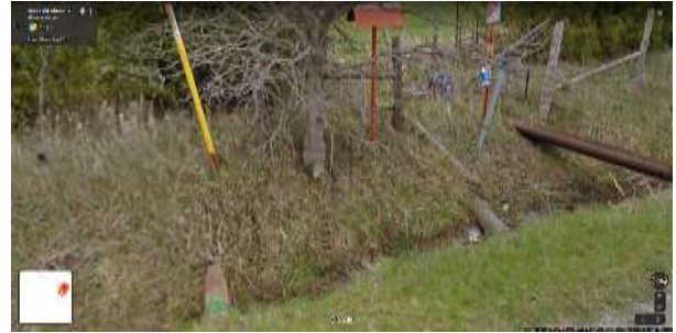
Figure 5.2-28: Exposed Ditch Crossing
