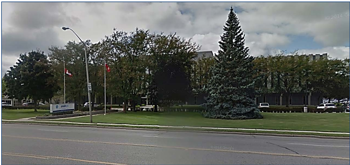
Figure 3.8: Union Head Office, 50 Keil Drive North, Main Building Front
