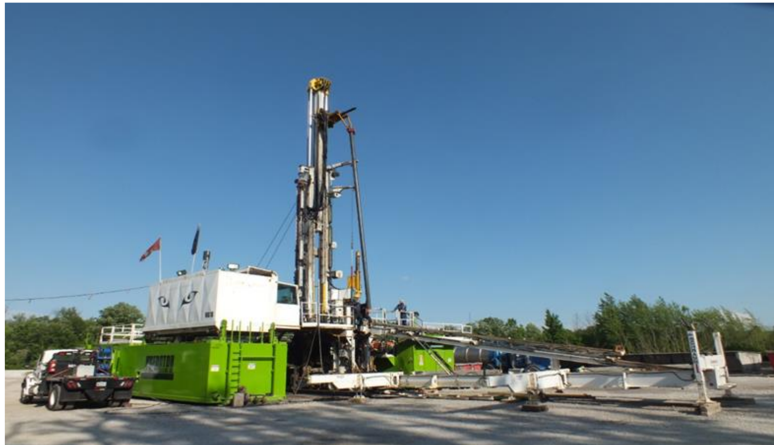
Photo 1. Photo of typical well drilling equipment
