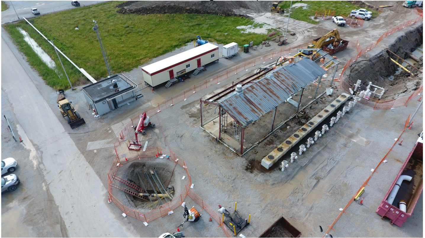
Measurement Building Removal (June 2023)
