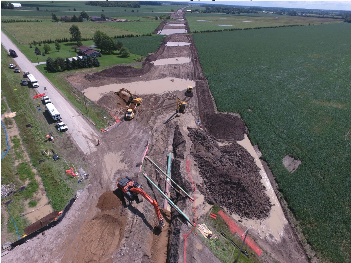
Wet soil shutdown following striping of topsoil (August 2023)
