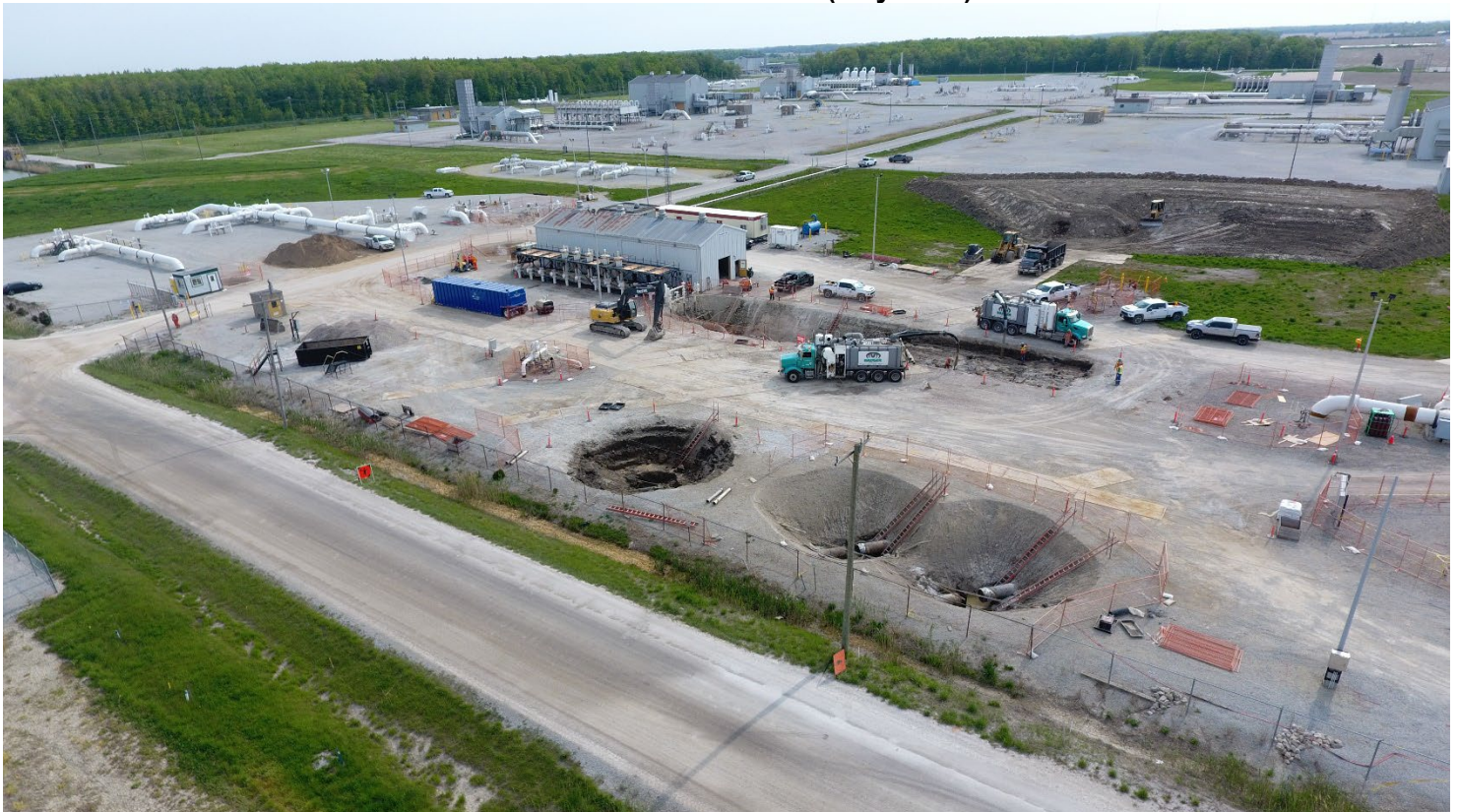
Dawn North Excavations (May 2023)
