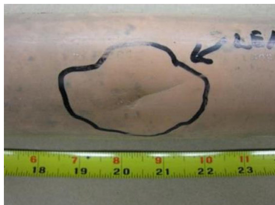
Figure 5.2-59: Sample of Aldyl-A Pipe with Crack Failure
