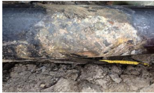
Figure 5.2-54: Coating damages
