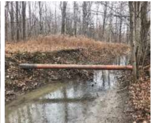
Figure 5.2-30: Exposed Crossings
