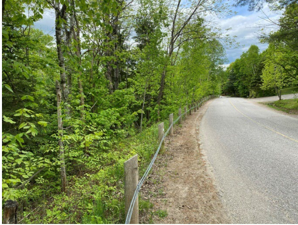
Photo 9: Steep embankment, slope in excess of 20°, looking east along Skyline Drive
