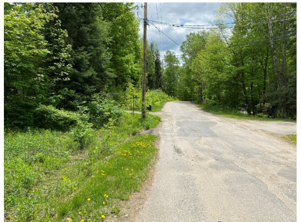
Photo 20: Previously disturbed right of way associated with road construction and ditching along shoulders, looking south
