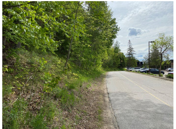
Photo 32: View of study area along Valley Road, looking east, with area of disturbance on the right and slope in excess of 20° on left
