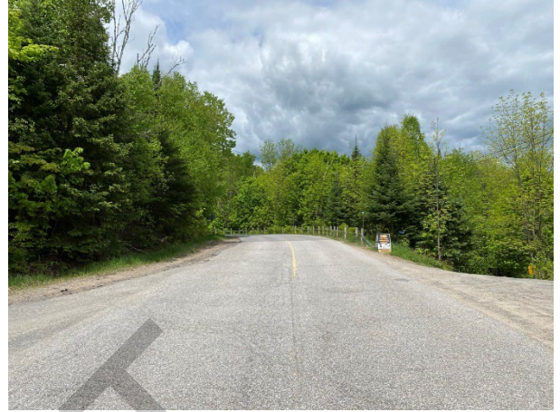
Photo 10: Steep embankment, slope in excess of 20°, looking northwest along Skyline Drive
