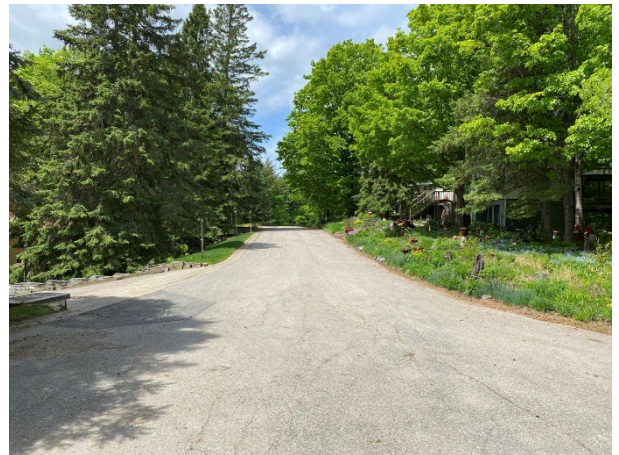
Photo 12: Previously disturbed right of way associated with road construction and ditching along shoulders, looking west
