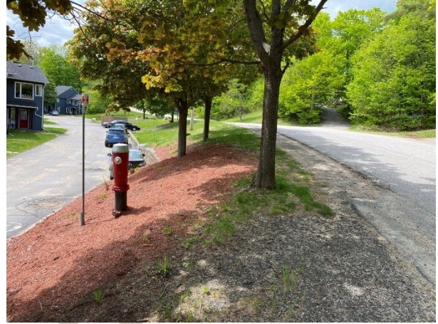
Photo 6: Steep embankment, slope in excess of 20°, looking east along Hidden Valley Road
