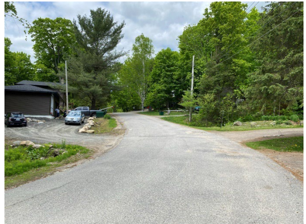
Photo 16: Previously disturbed right of way associated with road construction and ditching along shoulders, looking northwest
