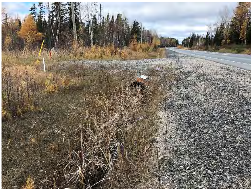
Photo 6: Disturbed area due to grading, ditching and installation of road and culvert – not surveyed, facing north
